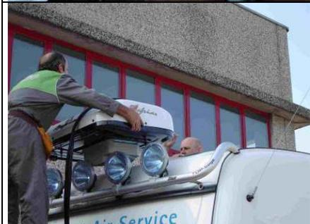
10. Place the TopCooling on the roof of the cab and guide it through the hole in the roof.
