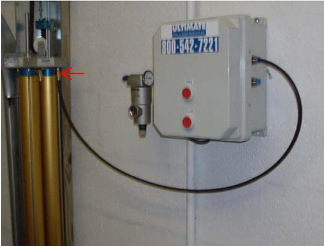
3. Connect bottom port of control box to elbow on cylinder farthest away from wall. ( See below)
