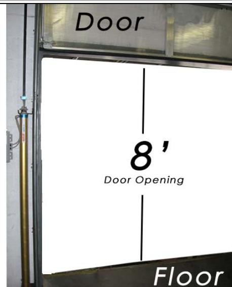
Rod with turnbuckle (Part No. CL100 and CL101) will rise when opening the door
