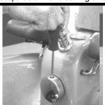
To remove the chrome drain handle, loosen the set screw in the slot on the drain handle and slip off chrome handle from chrome handle post.
