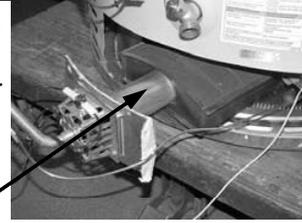
Step 9. Remove the pilot assembly from the main feedline using a 1/4" nut driver.
