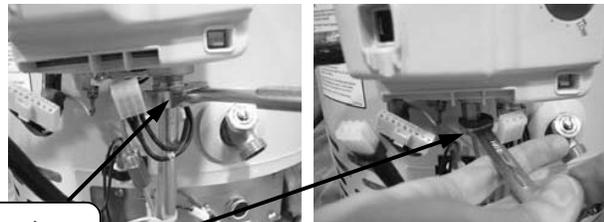
Step 7. Disconnect the spark igniter/flame sensor wire from gas control.
