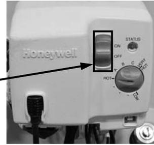
Step 1. Move the gas control power switch to the "OFF" position.
