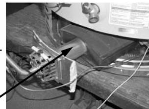
Step 10. Remove manifold mount from burner inner door by removing (2) 1/4" hex drive screws.
