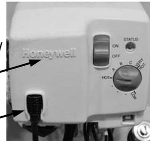
Step 6. Using the gas control service tool, p/n 239-45991-00, available from your BWC parts supplier, insert the tool into the back of the gas control.
