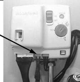
Step 3. Using a multi-meter set to the ohms setting, measure the resistance of the flammable vapor sensor and resettable thermal switch. The resistance must be between 3,000 and 48,000 ohms. If the resistance is out of this range, verify that the resettable thermal switch has not been tripped. If it hasn't, replace the thermal switch.
