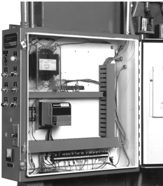
Fig. 7. Electrical panel installation.
