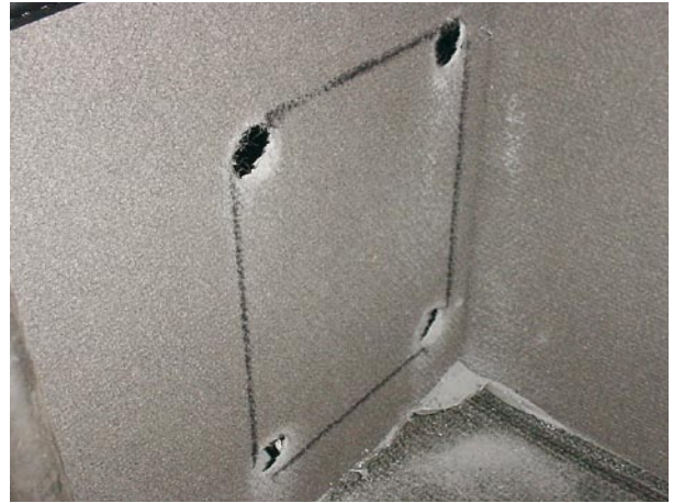
Figure 8 - Location for cutting return air vent
