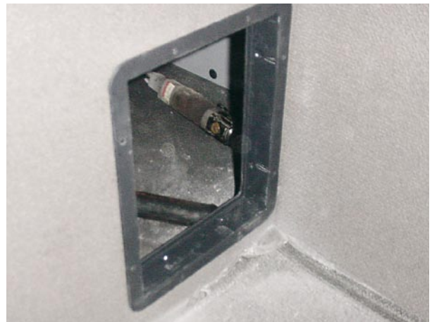
Figure 10 - Return air grill flange installed
