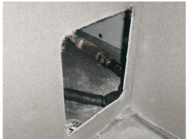
Figure 9 - Return air vent hole cut
