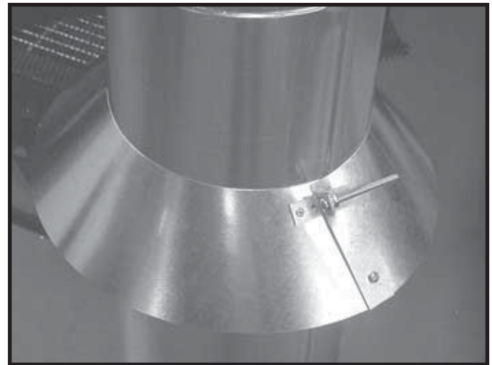
Figure 8.17 Assembling the Storm Collar Around the Pipe
