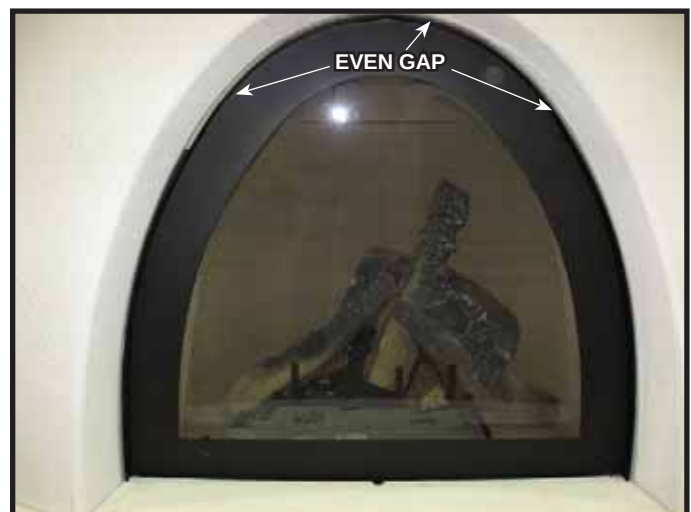
Figure 11.11 Even Gaps All Around.
