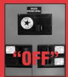
**NOTE: Balance must be maintained when moving circuit locations from main electrical distribution panel to emergency load center. Circuit breaker positions alternate buss bars vertically. Circuits sharing a neutral wire should either be moved together to adjacent positions in emergency load center or not moved. If you are unsure of proper procedure or if your installation differs from that described in this guide, consult a licensed professional at this time.**
