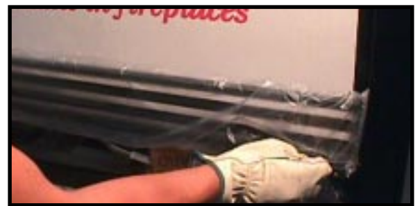
Figure 20 - Control Access Panel Removal
