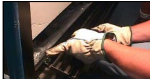
Figure 23 - Replacing the Control Access Panel
