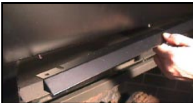
Figure 18 - Hood Placement
