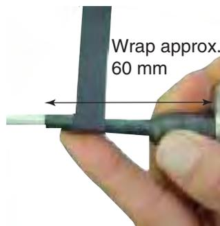
2. Completely cover the butyl rubber tape with white vinyl tape, wrapping from the base to the last wind of butyl rubber tape and then back to the base.
