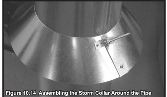
Figure 10.14 Assembling the Storm Collar Around the Pipe
