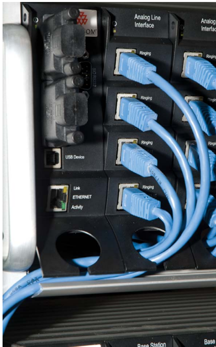
Figure 1-9 Harnessing cables to the side and out.
