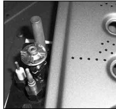
**Figure 7. Ignitor assembly beside the burner.**
