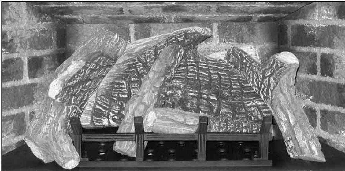
**Figure 27. Third Stage Log Set Installation.**
