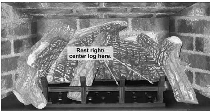
Figure 26. Second Stage Log Set Installation.
