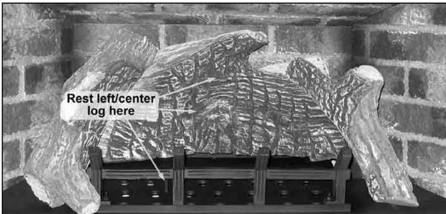
Figure 25. First Stage Log Set Installation.
