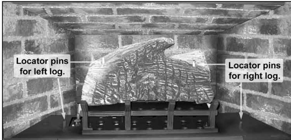
Figure 24. Empty firebox with grate and locator pins.
