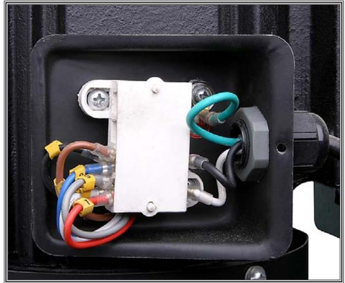
Figure 35. Motor junction box wiring.
