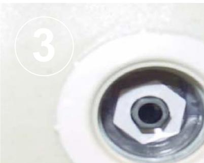
Remove the jet nozzle and nut using a 7/8" deepwell socket and extension.
