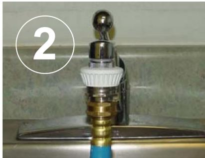
Screw the white quick connect adaptor into the blue female hose. Connect the adaptor to the faucet by sliding the white sleeve down while sliding the connector onto the faucet adaptor.
