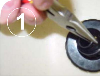
Remove the jet eyeball using the needle nose pliers.
