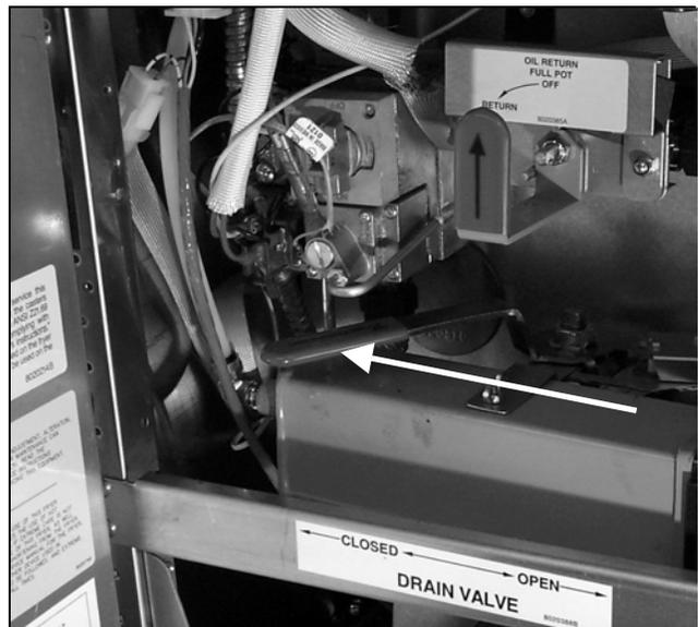
7. Let the filter run 10 to 12 seconds after oil/shortening stops coming out of the Power Shower to clear the lines and prevent shortening from hardening in them. Rotate the oil return handle to the OFF position to stop the pump. Remove the Power Shower and allow it to drain. Turn the fryer on and allow the cooking oil/shortening to reach setpoint.
