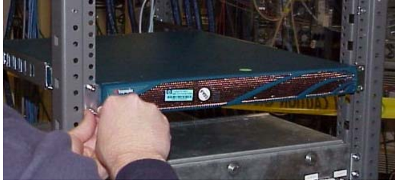
Figure 1-6: Secure switch with screws through the front of the rack
