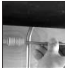
Completely insert dispenser faucet copper tube (marked with white tape) into the quick-connect union fitting.
