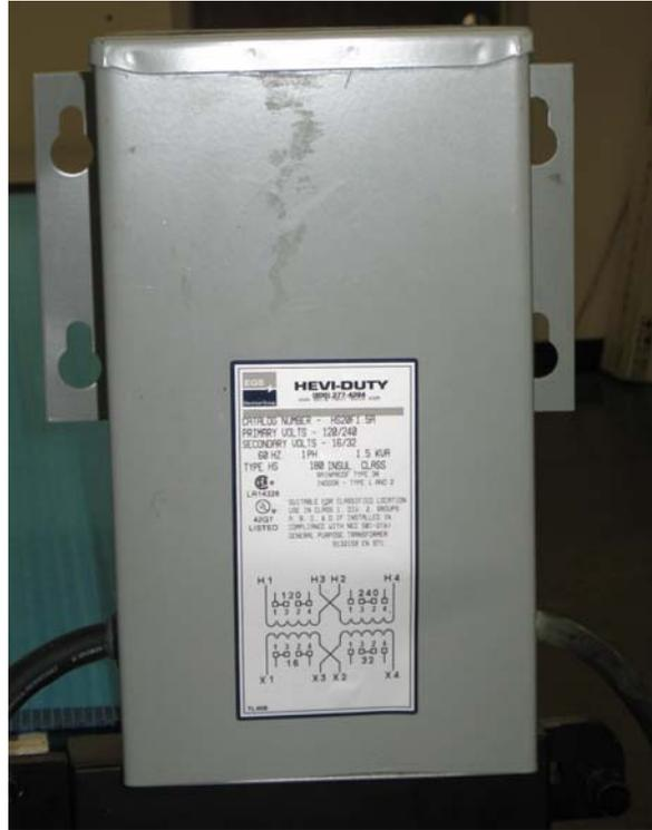
This photo is showing a sample Buck Boost Transformer from Sola Hevi-Duty, it is a 1.5 KVA version, catalog # HS20F1.5A and it weights approximately 38 pounds or 17.2 Kgs.
