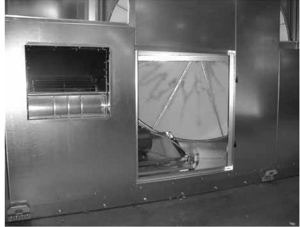
FIGURE 26: Access to wheel through exhaust blower door.
