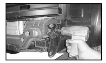
**12.** Remove tie down brackets from each side, three bolts from each side, these will not be reused.
