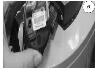
Step 6. Reconnect wires from step 5 to new pressure switch.
