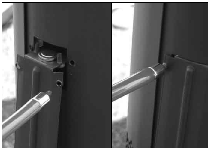
Figure 43: Spill switch installation.
