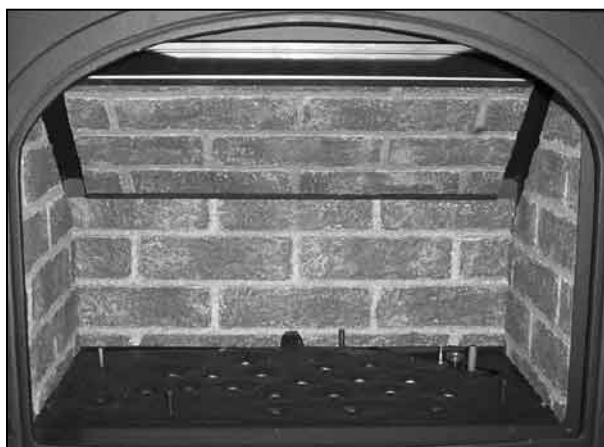
Figure 59: Side brick panels in place.
