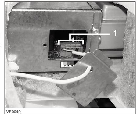
10. Reinstall the side door on the electrical box.
