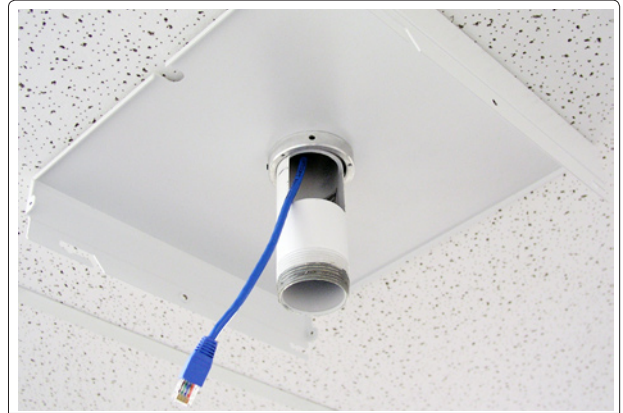
4c Run the cable(s) through the projector pole.
