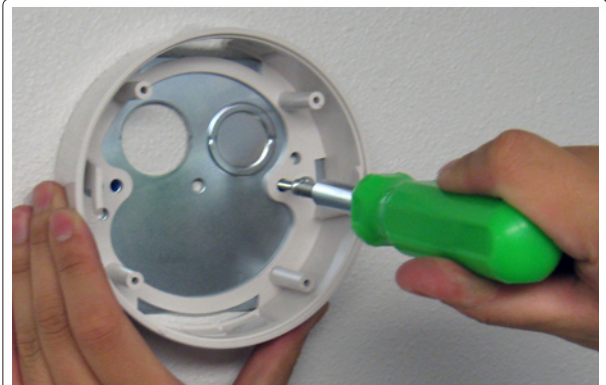
4a Mount the receiver housing to the mounting surface using screws.
