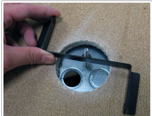
②b Attach the Z bracket loosely to the ceiling tile and the back plate.
