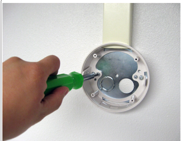
4b If using a raceway, insert the raceway through the knockout, then mount the housing.
