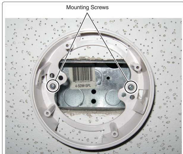
②b Attach the receiver housing to the junction box.
