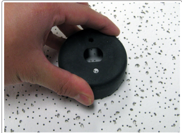
①b Cut a hole in the ceiling tile.
