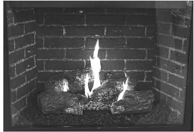
**Figure 52 - Burner Flame Appearance Model SLDVT-40**
