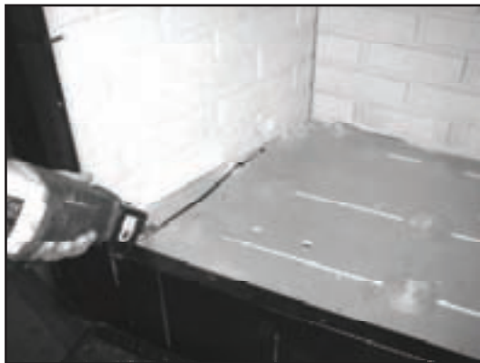
Figure 11.2. Using a saws-all, cut out the floor
