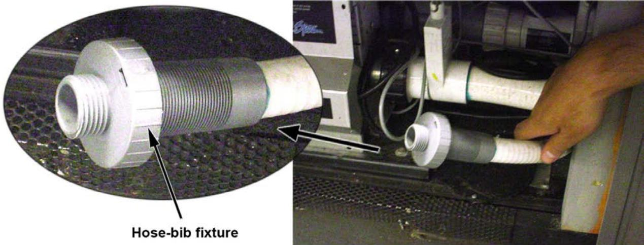
5. Hook up the female end of a garden hose to the drain fitting.
