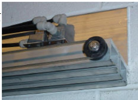
**21** Continue running cable around bottom of pulley on left side of track. Connect cables together in center with turnbuckle.
