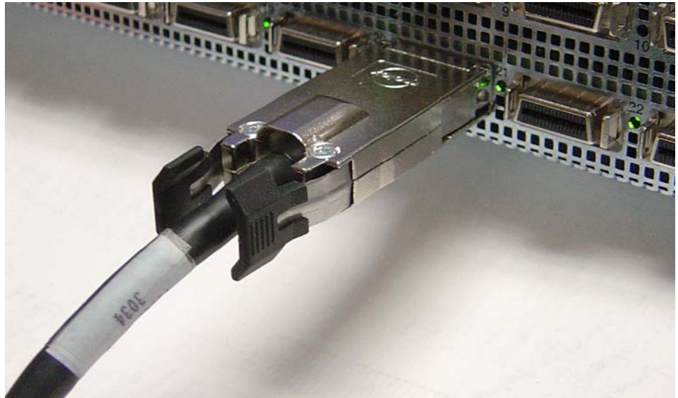
Figure 1-7: Fully Installed IB Cable with Pinch Connector
