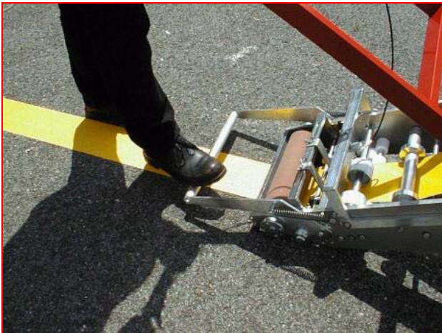
Figure 10: Cutting the tape
