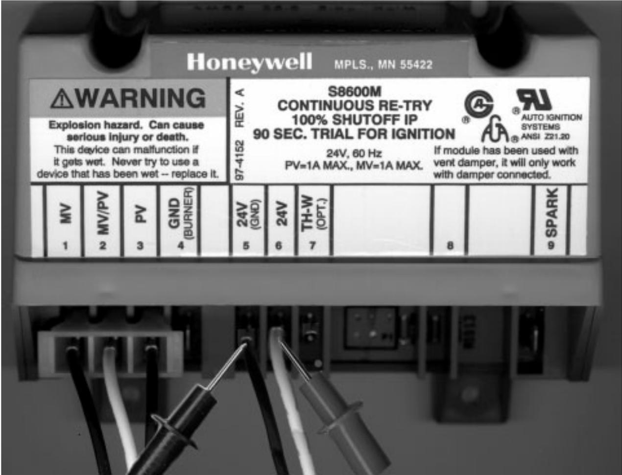
**STEP 11. WIRE HARNESS TEST.** Test for 24 VAC between terminal 24V on the IID module, and 24V GND.
