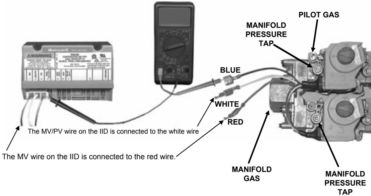
**STEP 14B. PILOT VALVE TEST – SBD 500 ONLY.** Testing the two coils of the Honeywell VR8404P 5004 gas valve used on the model SBD 500 only. Because of built in diodes, it is difficult to test for ohms resistance through these coils. The following is a DC amperage check of the main and pilot coils.
