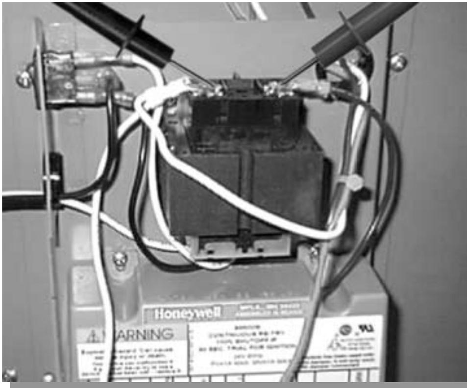
**STEP 1 - TO TEST THE TRANSFORMER** - Using a multimeter, test for 24 VAC between the secondary transformer terminals.
