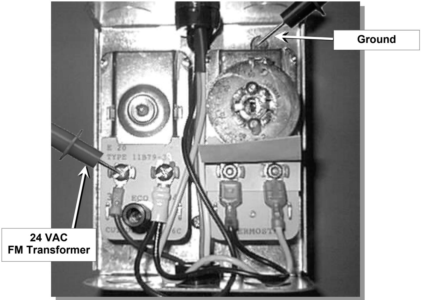
**STEP 2. HIGH LIMIT, LEFT TERMINAL TEST.** Test for 24 VAC between the left high limit terminal and ground.
