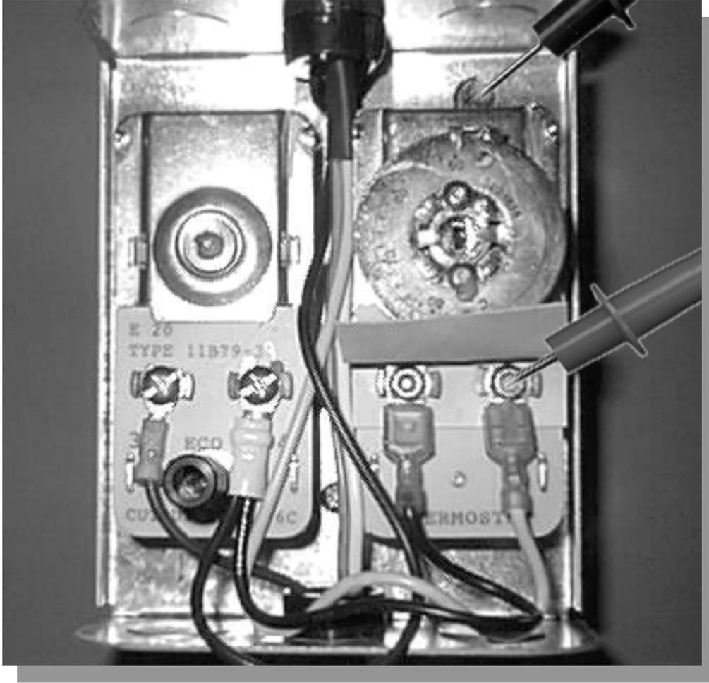
**STEP 7. THERMOSTAT TEST.** Set the thermostat to call for heat. Using your multimeter, test for 24 VAC between right terminal and ground.
