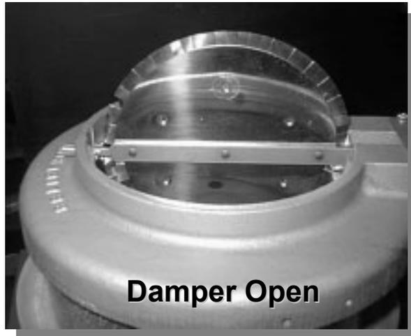
**STEP 4. INSPECT THE DAMPER.** Lower the thermostat setting so the unit will not be calling for heat, then inspect the damper.
