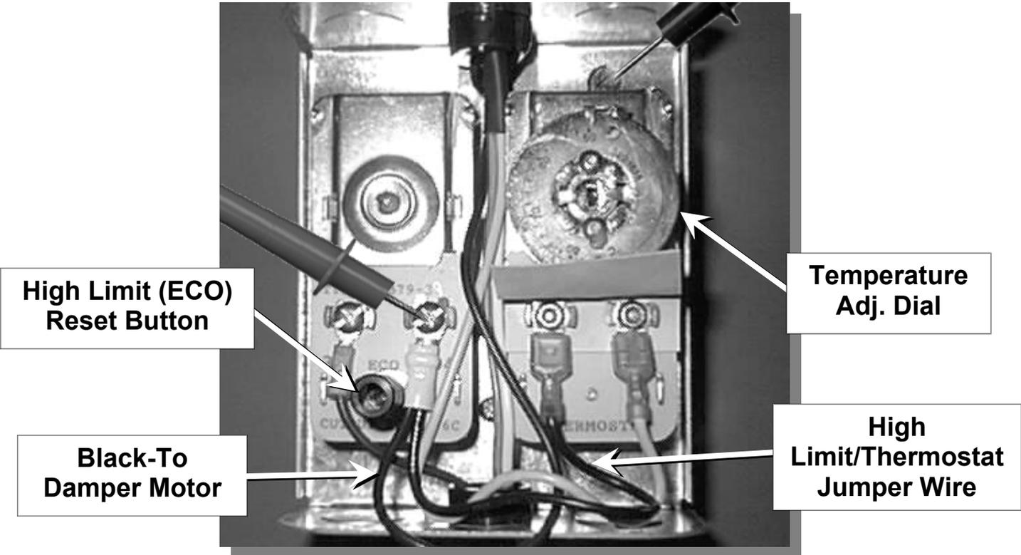
**STEP 3. TO TEST HIGH LIMIT RIGHT TERMINAL.** Ensure that the jumper wire between the high limit and thermostat is connected, and the damper motor power line is connected. Test for 24 VAC between the high limit right terminal and ground.
