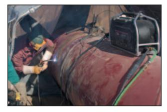
feedability and excellent arc characteristics, a result of Lincoln's manufacturing which uses a strictly controlled chemistry process. All mainline welds are inspected using automatic ultrasonic tests.
