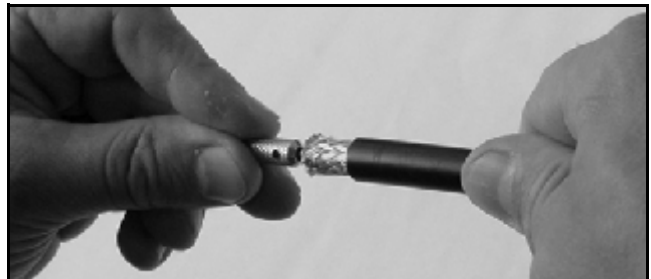
Figure 56: Deburring the Center Conductor
