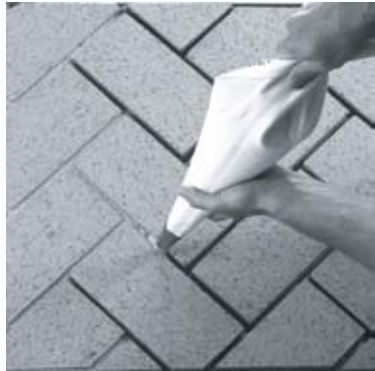
Figure 20 - Grouting Brick INSTALLING SCREEN
