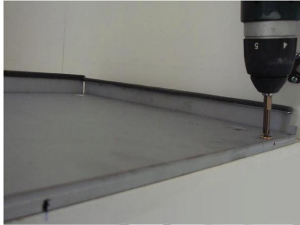
1. The cavity must be made to the specifications set out in Sharp's kitchen cabinetry requirements for built in microwave ovens. Mark the centre of the cabinet base panel. Sit the Base Assembly into the kitchen cabinet and align the base centre alignment cut with the centre mark you have just marked on the cabinet base. Ensure the front edge of the trim kit base is flush with the front edge of the cabinet base front edge. Use the 2 button head screws provided and screw into position.
