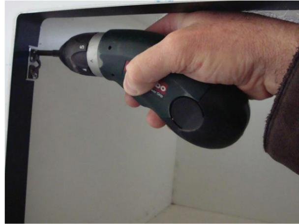
2. Position the Fascia Assembly into position with the female clips attached correctly. Once it is in its correct position (see Cabinet Specifications in this manual), screw the female clips into position using the 6 gauge screws provided.
