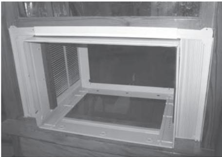
**NOTE:** Do not shut the window so tightly that movement of the accordion panels is restricted.
