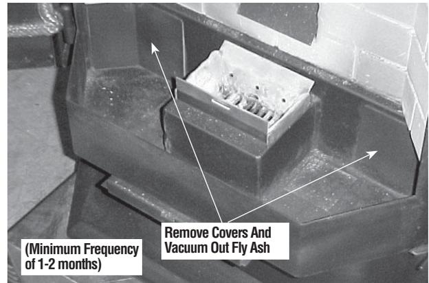
**Figure 43 - Accessing Ash Clean-Out Ports – Profile 30 Series**
