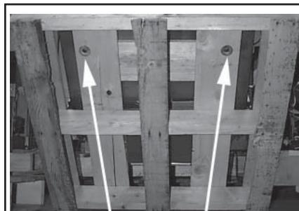
Remove the three bolts from underneath the pallet.
