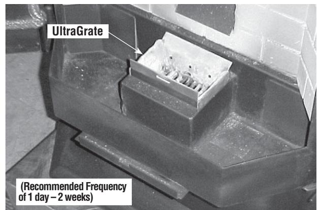
**Figure 44 - Inspect UltraGrate and Clean if Necessary**
