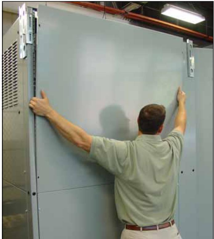
Figure 41. Lifting the Cover Free.
