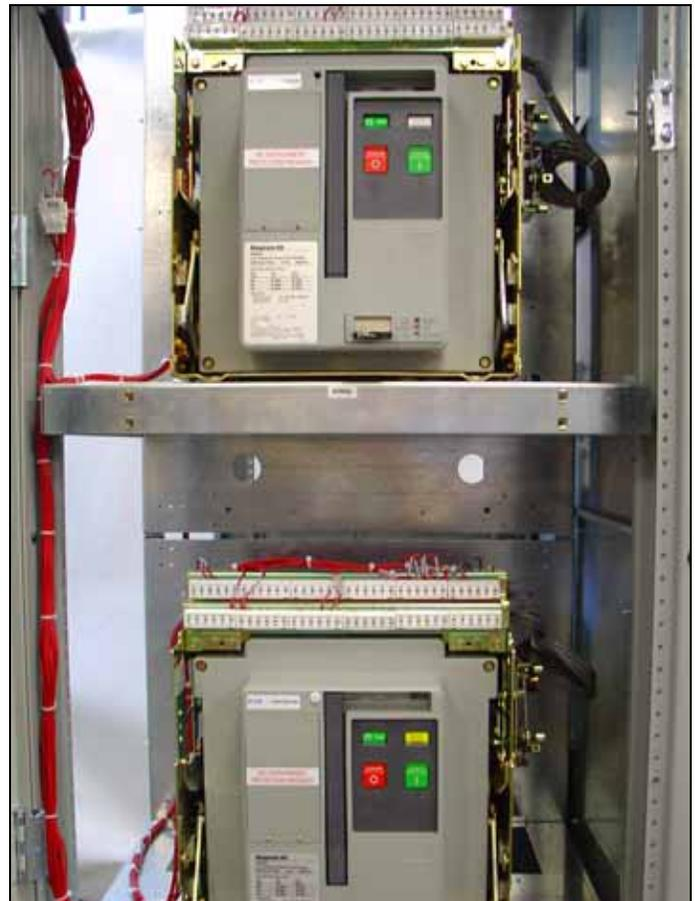
Figure 11. Typical Power Panel (Open Transition Shown).
