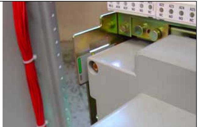
Figure 31. Switching Device in the DISCONNECT Position.
