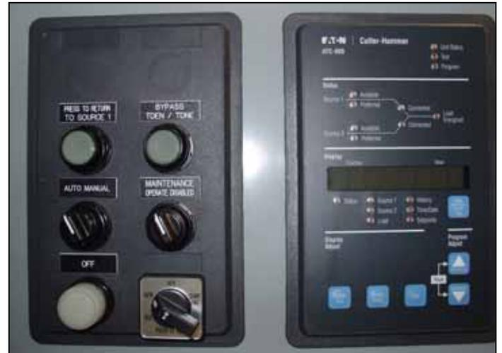
Figure 35. Bypass Isolation Switch.
