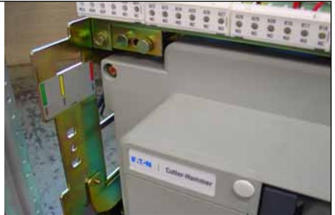
Figure 29. Switching Device in the CONNECT Position.
