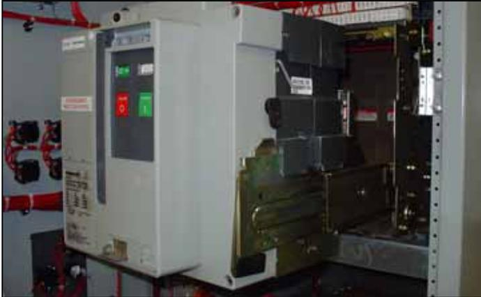
Figure 14. Drawout Mechanism (Closed Transition Shown)
