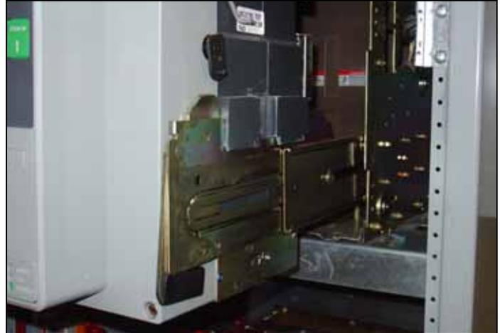
Figure 28. Switching Device in the REMOVE Position.
