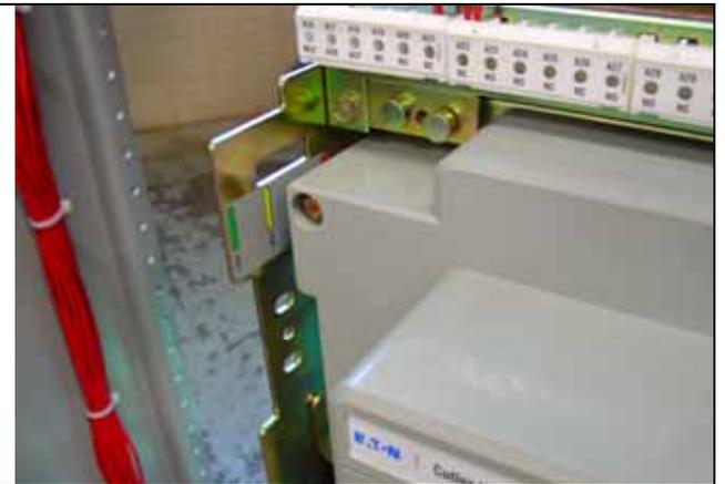
Figure 30. Switching Device in the TEST Position.
