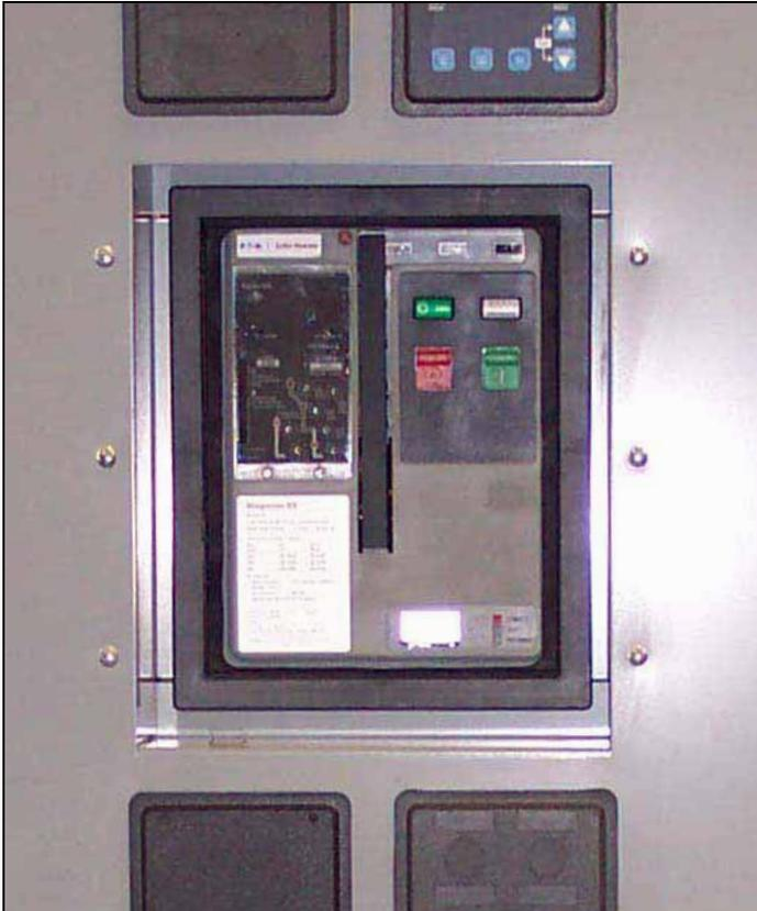
Figure 12. Insulated Case Switching Device.
