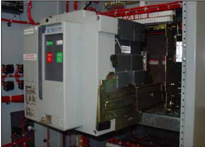
Figure 26. Switching Device Drawn Out from the Transfer Switch.
