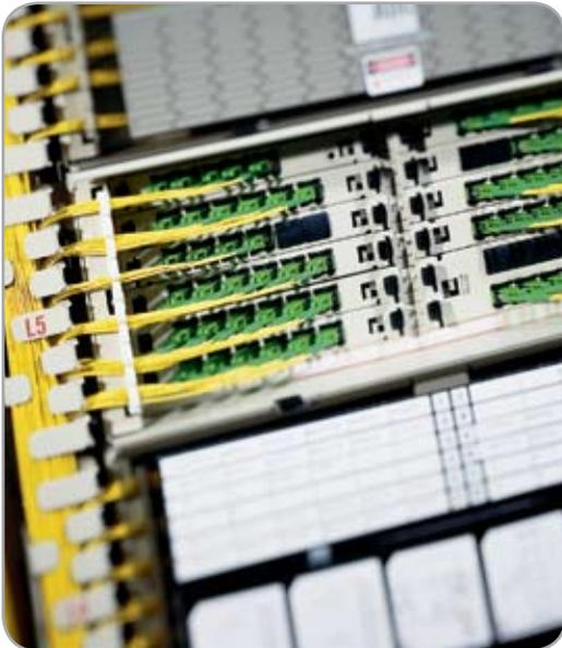
One-stop-shop for complete optical transport system support requirements. The VAM System consists of a variety of chassis and value-added modules housing various optical components that fit into existing ADC fiber distribution frames and along with various other mounting environments.
