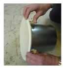
Loosen the four attachment screws and fold the tabs sideways until they touch the steel back can, allowing the speaker to pass freely through the cutout. Assemble the speaker, tile bridge and tile together and tighten the attachment screws to tighten the mounting tabs. Note that the first 1/4 turn rotates the tab outwards and away from the can, and subsequent turns tighten the tab down onto the ceiling tile. DO NOT OVERTIGHTEN.
