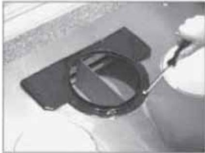
1. Remove pre-mounted 7" transition adaptor or duct opening.
