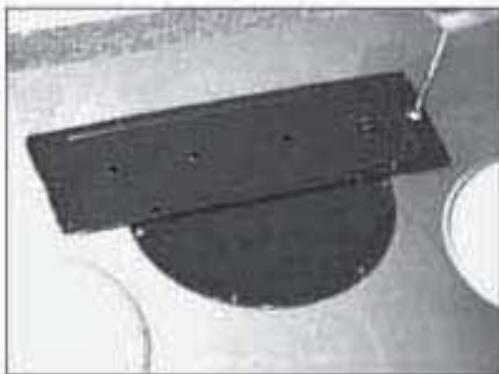
6. Mount rectangular cap (previously removed) on top of transition adaptor. Seal all open holes with duct tapes.
