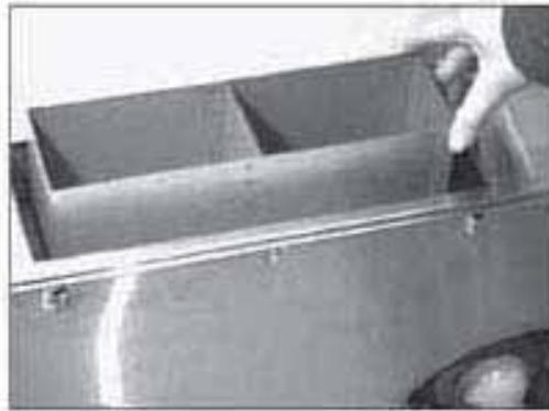
4. Mount starting collar (provided) at rear discharge opening with gasket previously removed.
