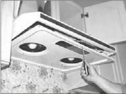
15. Next, fasten the 3 front screws and begin tightening all screws from rear to front.
