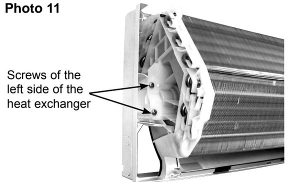
Screws of the left side of the heat exchanger
