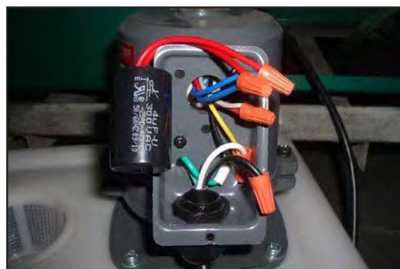
Figure 50. Pump motor wiring and capacitor (M2).
