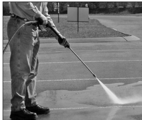
Figure 14 - Optimum angle to cleaning surface
