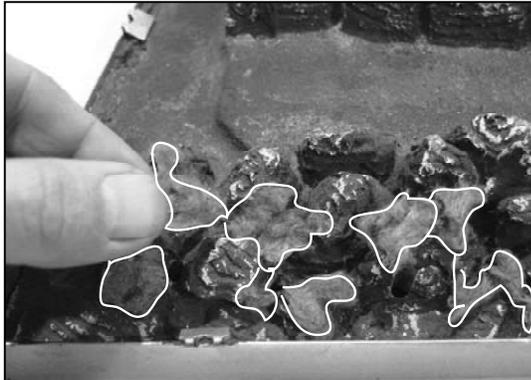
**Figure 8.21** Place individual pieces of embers in front of and around the gas log where they can be seen. Space them so that gas can contact them on all sides. Avoid stacking the embers on top of each other.
