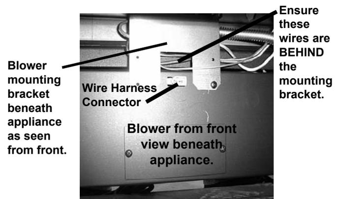
**Figure 8.23** Beneath the appliance from its front side, ensure that all wiring is moved behind the blower mounting bracket which already comes installed on the bottom of the appliance. Complete blower mounting by inserting two screws through the blower into the mounting bracket. Make the wire harness connection.
