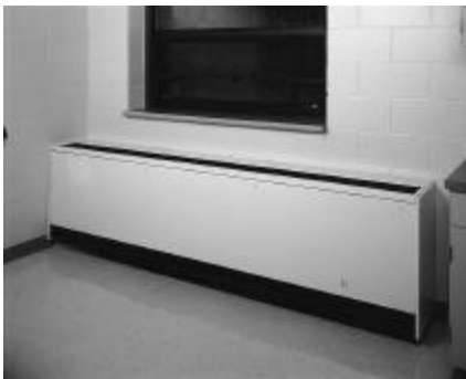
Figure 6: Typical classroom unit ventilator installation
