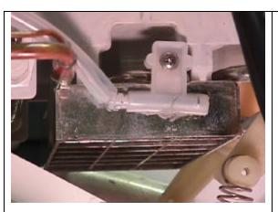
The freeze cycle is controlled by a thermistor, which is mounted at the evaporator outlet. The pump is spraying water up into the evaporator cells to form the square IM cubes. The evaporator temperature lowers as the ice cubes form.
