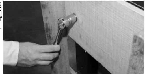
Removing skid from bottom of cabinet.
