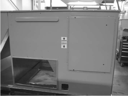
FIGURE 13 - SIDE PANELS WITH HOLE PLUGS
